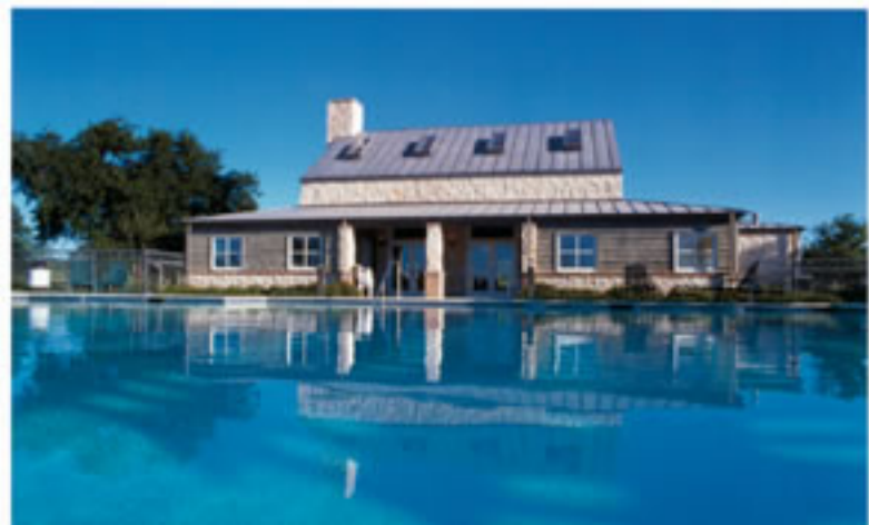
The Community Center with swimming, tennis and golf course located at the entrance of Coyote Ridge Development.
